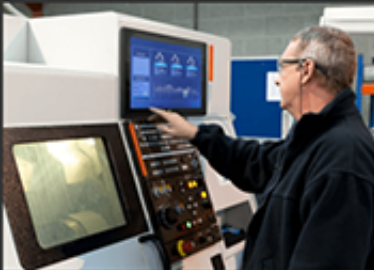
CNC Machine Operator Control Panel
